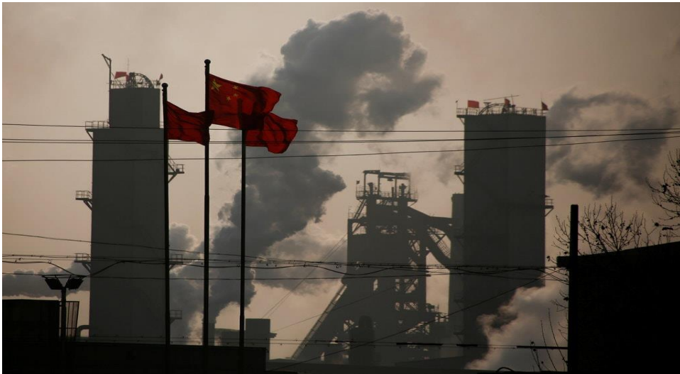
Figure 1: A steel factory in Wu'an, China. Many countries can report lower carbon emissions because they are increasing imports of materials like steel or cement. Credit...Thomas Peter/Reuters, Nytimes.
